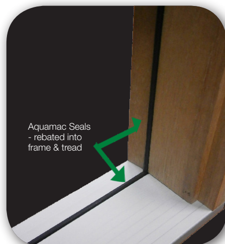
Contemporary aluminium, OPEN-OUT self-draining tread. 135mm x 35mm
