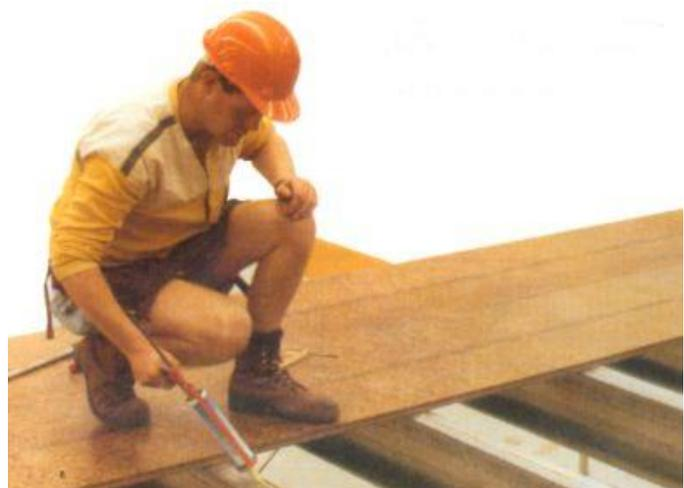
**Adhesive plus nails or screws is specified for the installation of all particleboard flooring.**
